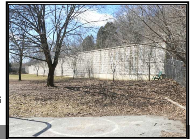
EXISTING WALL ABUTTING WATER FALLS
